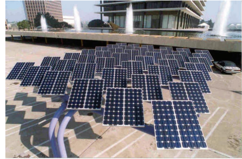
Fig. 2. One solar PV array cast shadow on another
