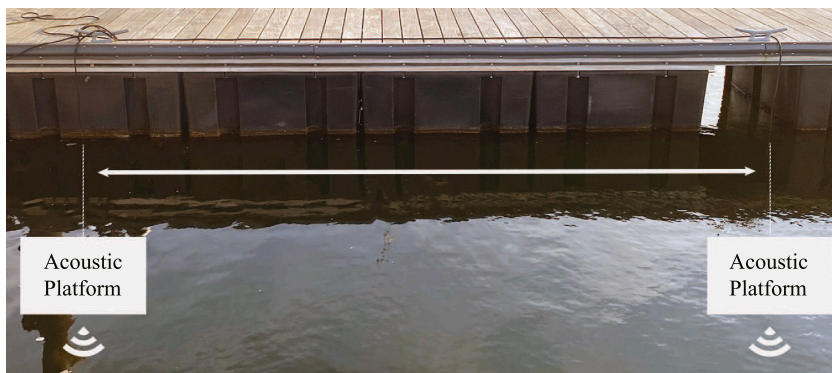
Fig. 8. Marina deployment setup.
